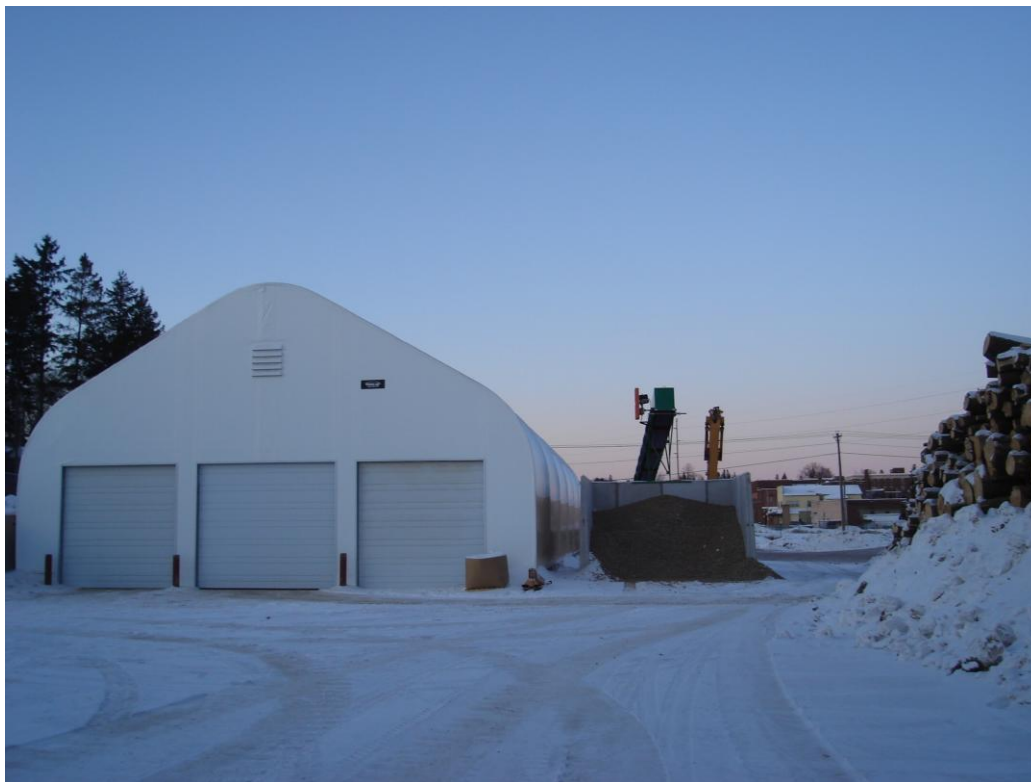
IMAGE 5: View of Densified Fuel Plant and Renewable Fuel Bunker (right of building) for No. 6 Boiler Fuel January 2009
