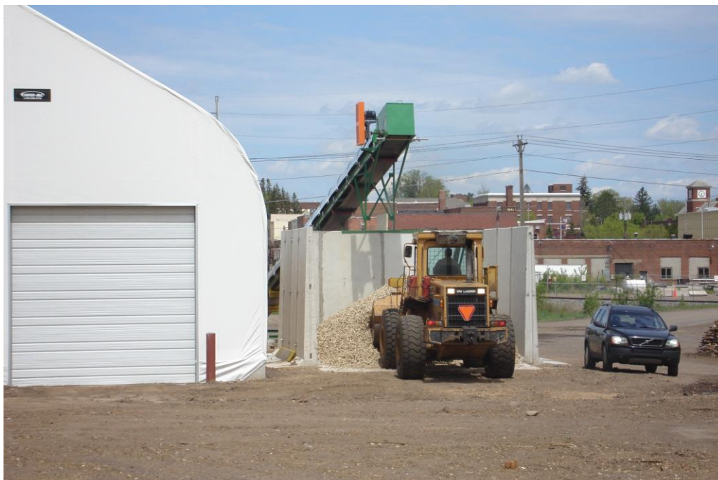
IMAGE 4: Front End Loader Retrieving Renewable Densified Fuel from Bunker at Flambeau Rivers Papers. LLC Park Falls, Wisconsin May 2009
