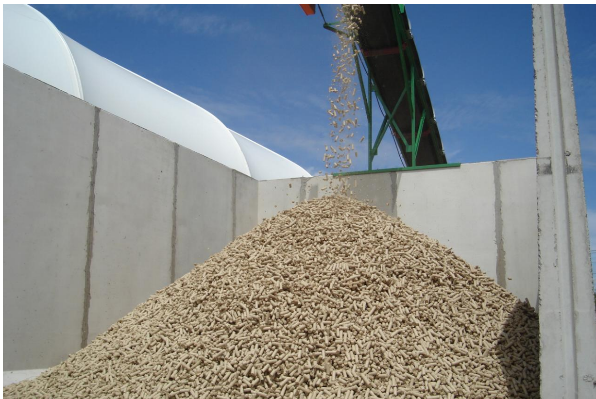
IMAGE 3: Outside Fuel Storage Bunker for Renewable Densified Fuel for No. 6 Boiler at Flambeau River Papers, LLC Park Falls, Wisconsin
