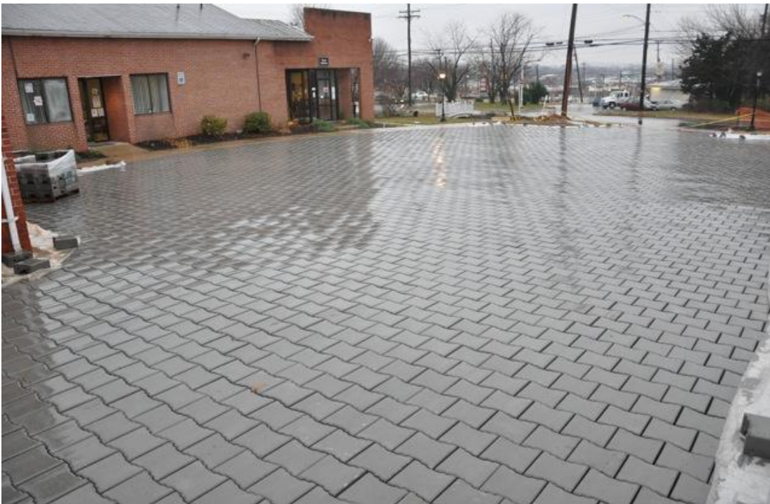
Finished installation of Bladensburg, MD Town-Hall parking lot.
